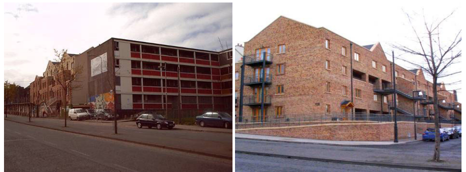
Bridgefoot Street – before and after refurbishment
