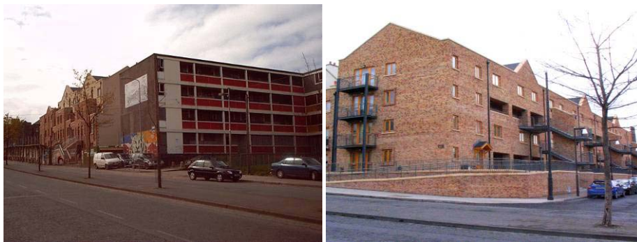
Bridgefoot Street – before and after refurbishment
