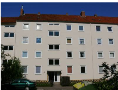
Demonstration project Euler Street in Hanover
